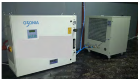
Figure 6. Ozone generator (Photo: B. Serdar Yıldırım)
